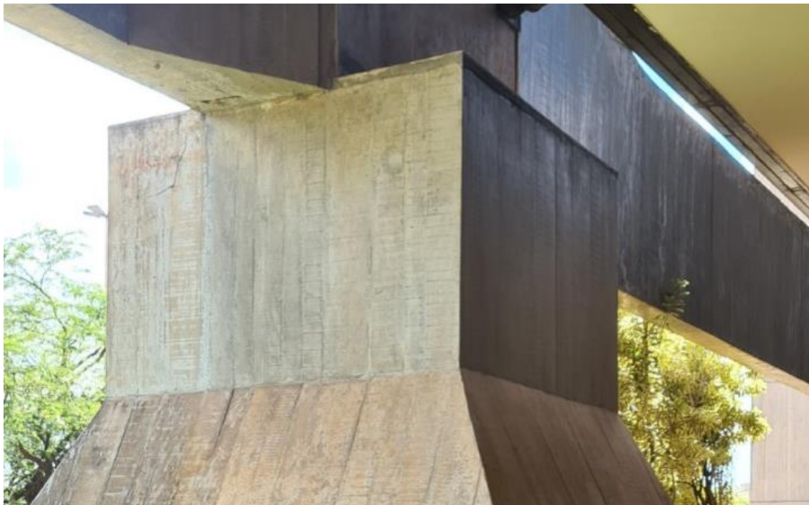
Figure 14 – Recovery and reinforcement carried out in the P4A pillar, after 15 years of execution.
